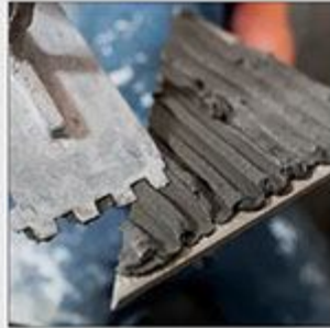
Cement Laying on Tile
