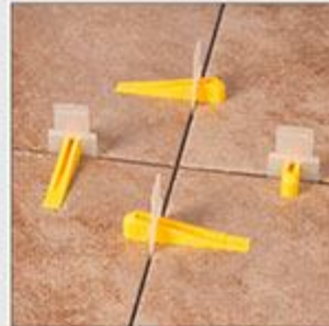
After Lavelling Process leave Int For 8-10 Hrs
