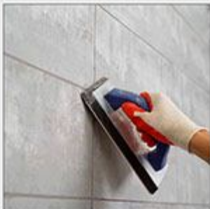
Joint Grouting
