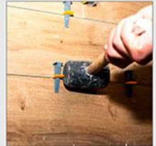
Remove Wedges Ones It Dry
