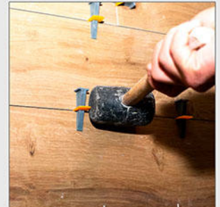
Remove Wedges Ones It Dry
