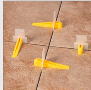
After Lavelling Process leave Int For 8-10 Hrs
