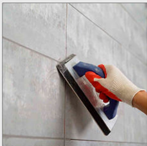
Joint Grouting
