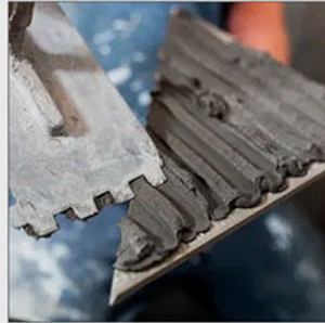
Cement Laying on Tile
