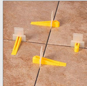
After Lavelling Process leave Int For 8-10 Hrs
