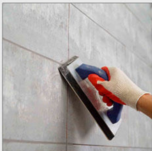
Joint Grouting
