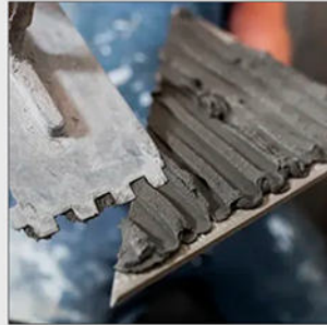
Cement Laying on Tile
