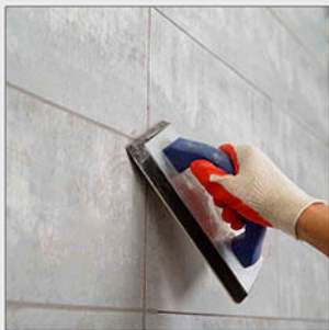
Joint Grouting
