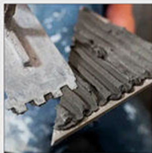
Cement Laying on Tile
